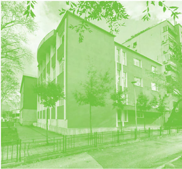
Secondary entrance to the “Jordan Misja” Lyceum through an extension in the form of a semi-cylindrical hall, photo by Jora Kasapi CC BY-SA 4.0.
