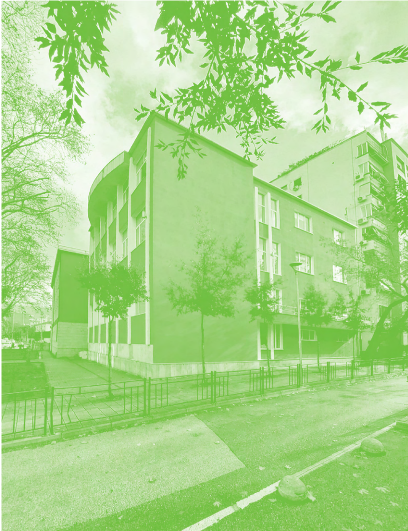
Fig. 8. Building extension for the visual art classes, constructed in the 1980s. Photo by Jora Kasapi CC BY-SA 4.0.
